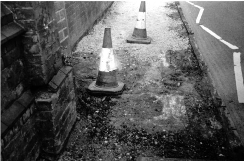
Photo 1. Concrete socket for tank barrier in Dunstable Street.
